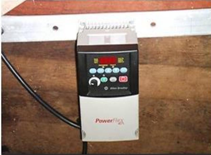
**Figure 5.** Shows the power supply to heat injection fan
