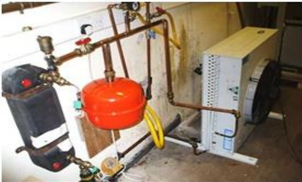
**Figure 3.** Shows the connections of the heat exchanger, water pump, heat rejection fan and expansion valve
