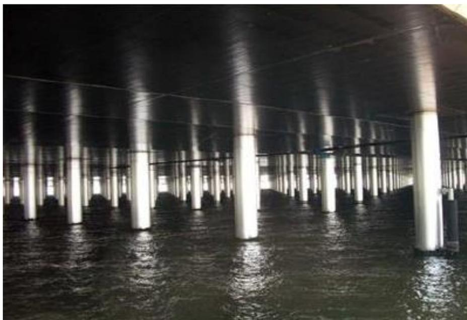
**Figure 6.** Pipe piles covered with stainless steel [8].
