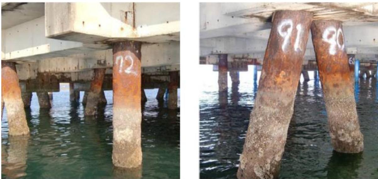
**Figure 5.** Corrosion-damaged pipe piles at an offshore pier [8].
