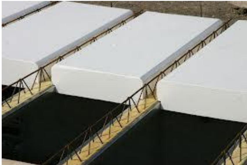
**Figure 6.** Ceiling of Styrofoam
