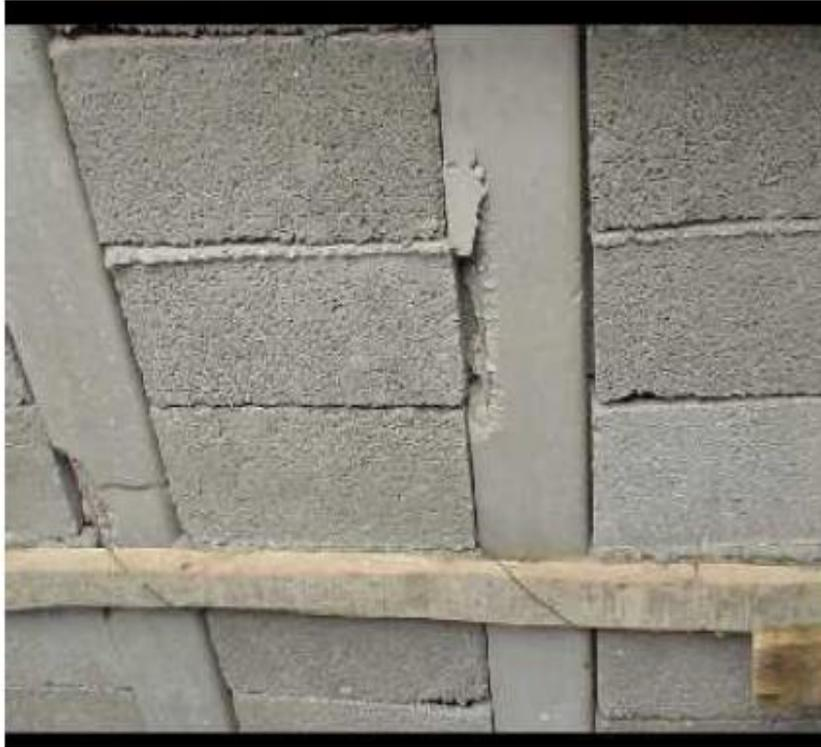
**Figure 4.** Damage to the heel concrete
