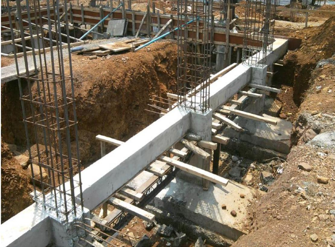
**Figure 2.** Individual footings connected by a plinth beam
