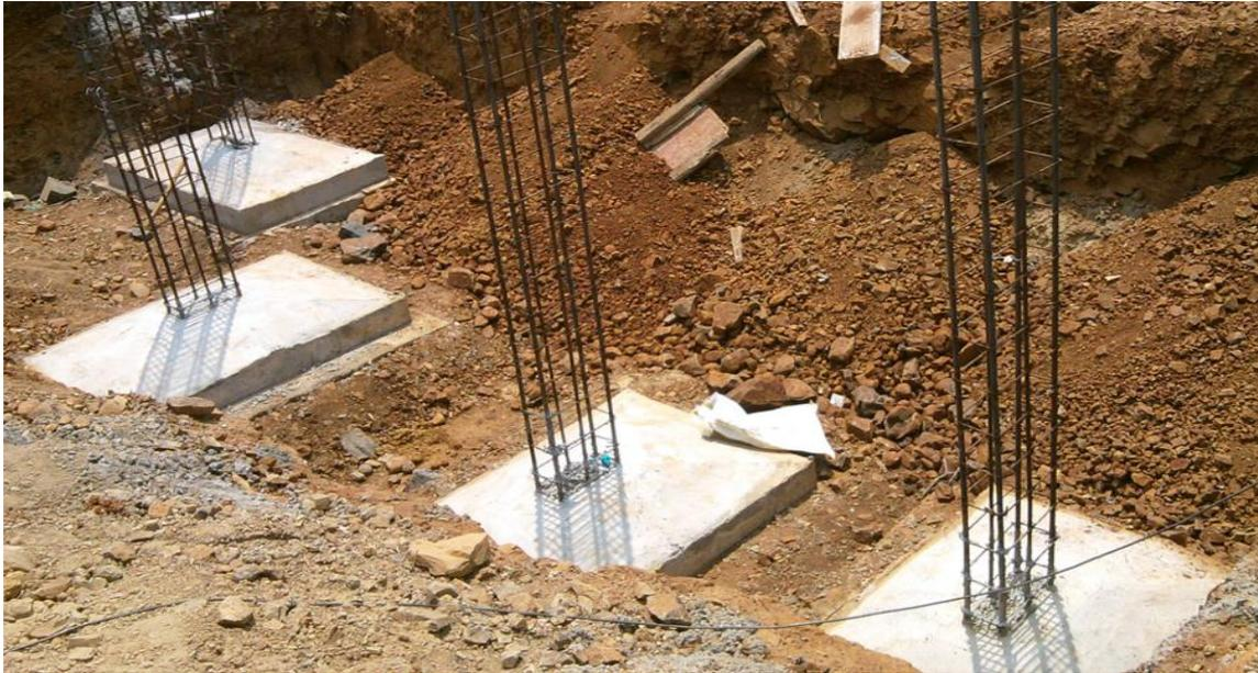
**Figure 1.** Individual footings awaiting concreting of the footing column
